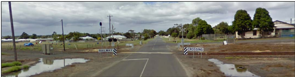
Figure 5: Cressy Road Looking East Towards Railway Level Crossing and Winchelsea Township
