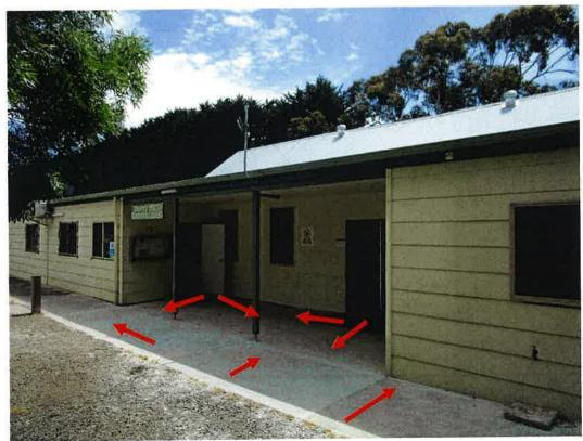
Photo 2; South of hall. Arrows show direction of paving fall.
