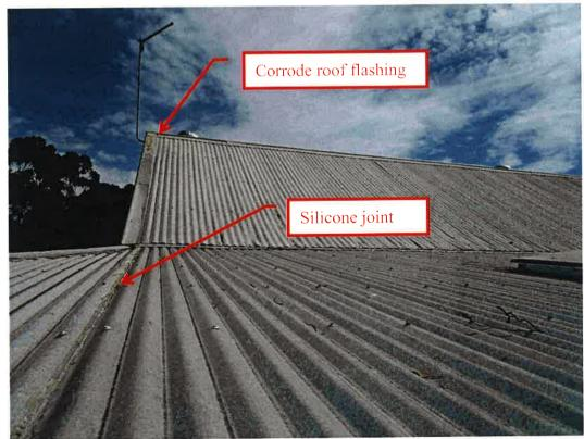
Photo 10; North side roof. Silicane joint. Corroded roof flashing.
