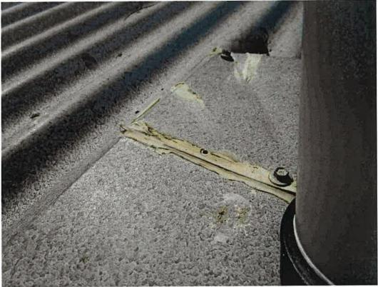
Photo 11; Example of poorly installed flashing. Missing roof screw and no pop rivits to hold sections together. Flashing not wide enough to extend to next corrugation fully. Screw at top not into top of corrugation.
