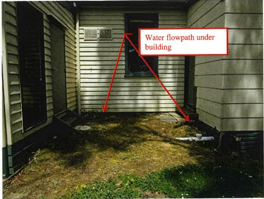
Photo 7; North courtyard; soil surface level higher than under building.
