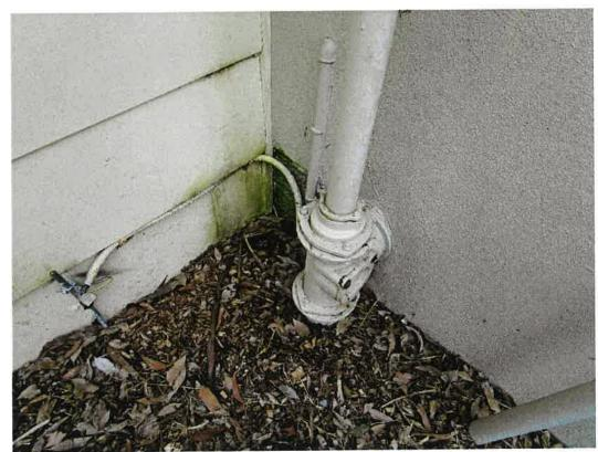
Photo 4; South east re-entrant corner. Algal growth indicating high moisture levels.
