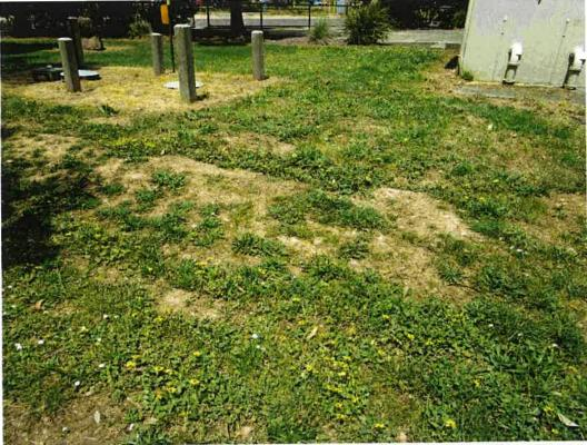
Photo 5; Septic tank location, within bollards. Uneven soil surface allowing for water ponding.
