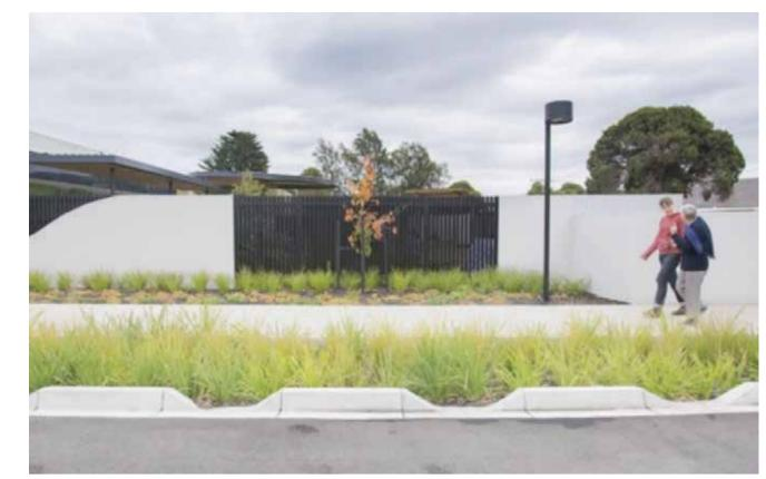
Kerb cut aways at proposed tree locations to enable passive irrigation
