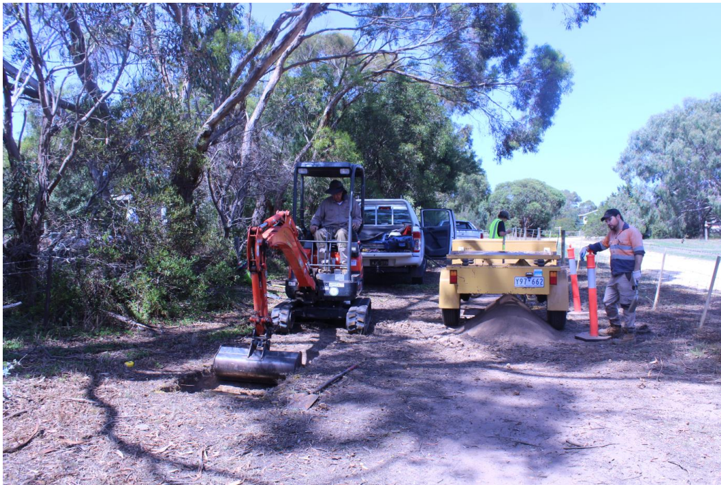
Figure 28. Mechanical excavations and sieving of mechanical test trench (MTT) 2.
