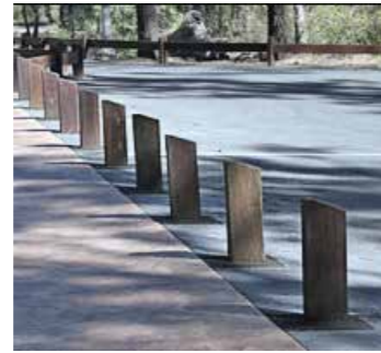
Indicative Vehicle Exclusion Bollards
