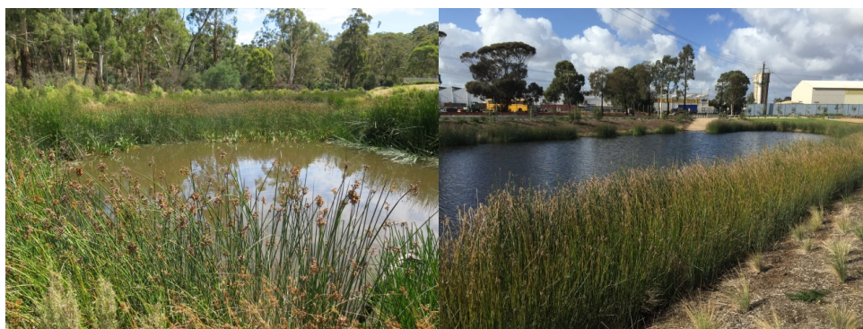
Figure 20 Examples of well established, vegetated sediment pond edges.
