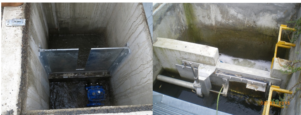
Figure 10 Examples of wetland controlled outlets: a) vertical slot weir, and b) sidewinding penstock valve (photo Melbourne Water).
