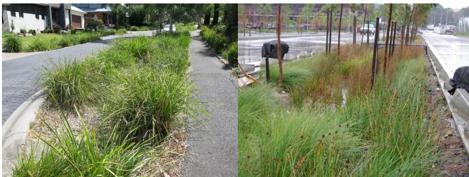
Figure 11 Examples: a) conventional swale, and b) bioretention swale.
