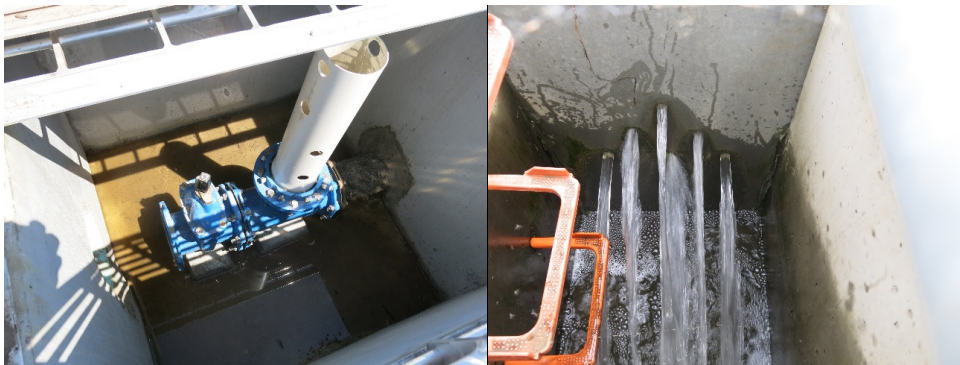
Figure 9 Examples of wetland controlled outlets: a) riser pipe, and b) weir plate.
