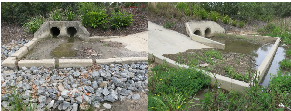
Figure 17 Examples of sediment forebays.
