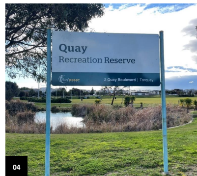
04 Large signage at Quay Reserve is mounted at a different height to other signs. Aluminium poles are used here instead of timber posts.
